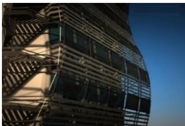
Figure 4: The Southern View of the Salehin Bank (Motahari, Tehran)
